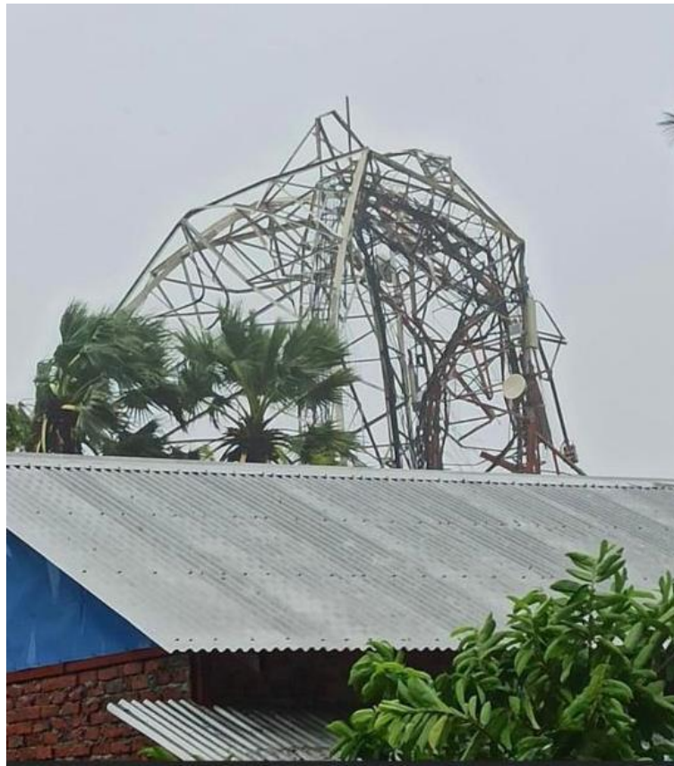
Figure 10. Telecommunications tower at Sittwe destroyed by Mocha
